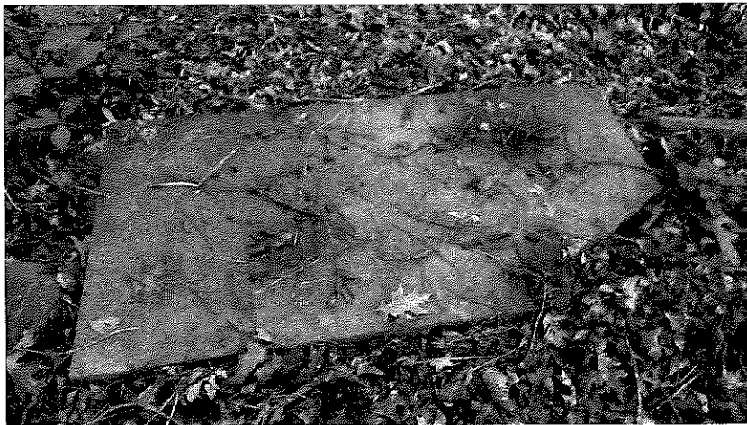
Ledger top panel missing corner
