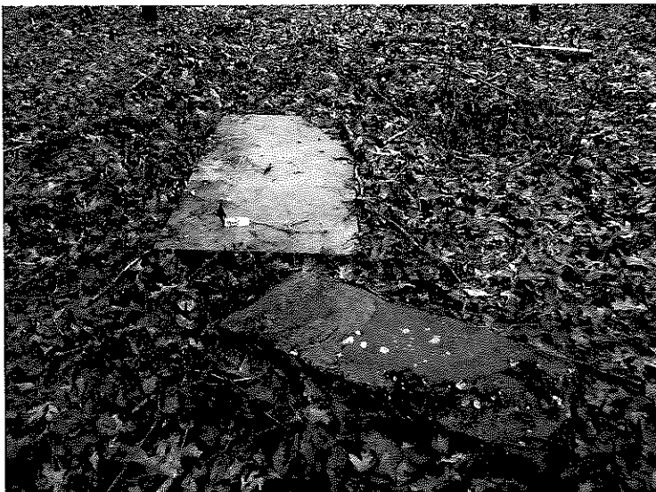
Collapsed ledger top and side panels
