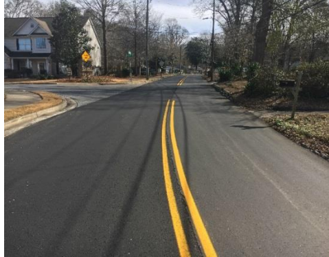
Northwest Drive Resurfacing
