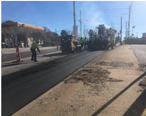
Metropolitan Parkway Resurfacing
