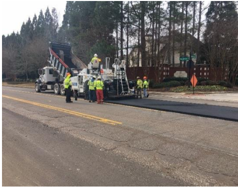
County Line Road Resurfacing
