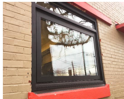
Atlanta Fire Rescue Station 23 Window Upgrades
