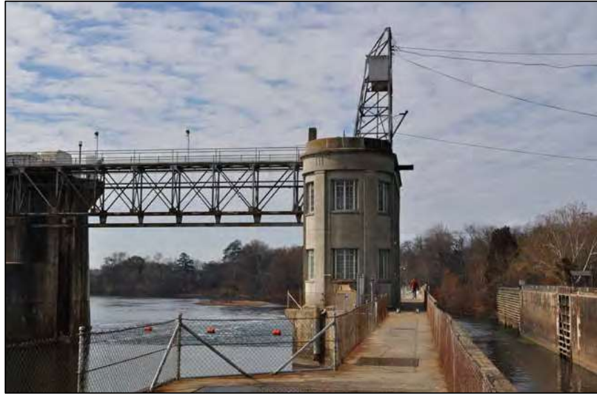
Figure 19: Operation Building Showing Relationship with Navigation Lock, Facing West (December 2012)
