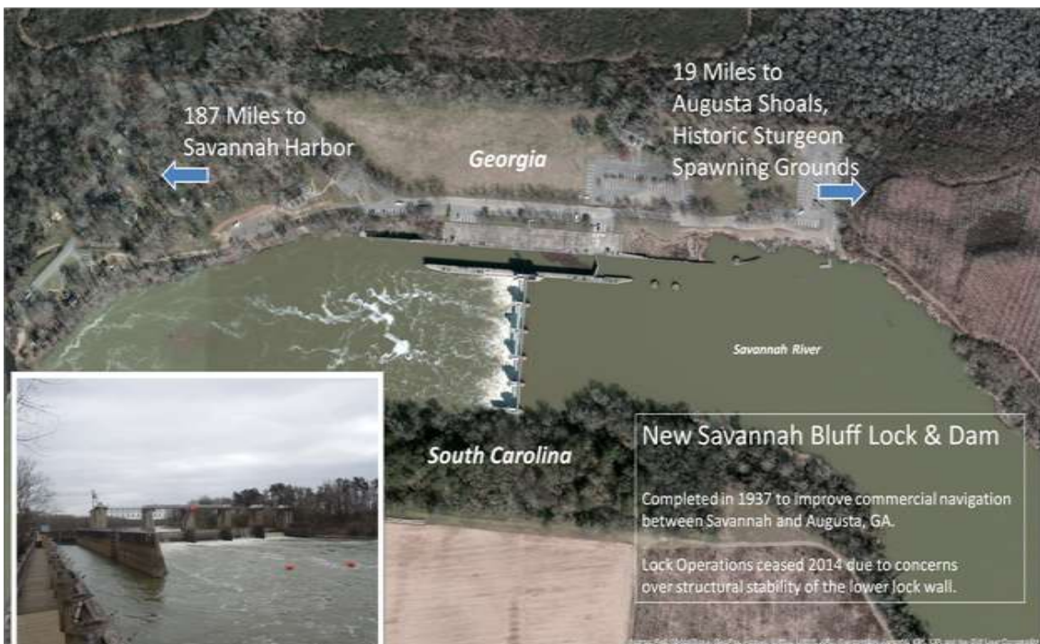
Figure 2: NSBLD Project Area
