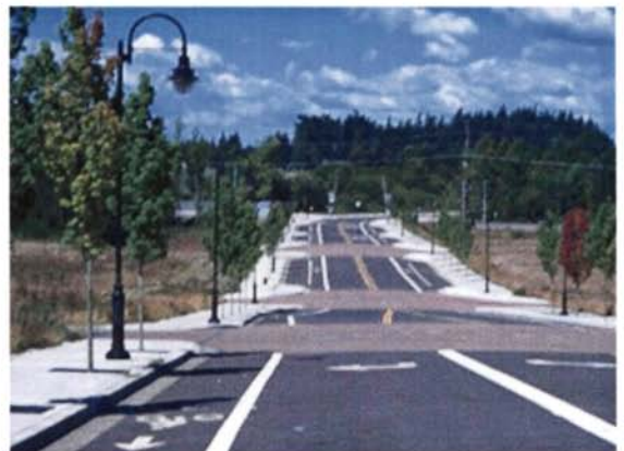
New infrastructure in Gresham with future rail stop
