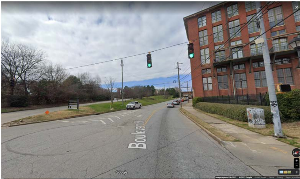
Figure 14. Street View image from NRHP Cabbagetown District towards proposed Hulsey Yard Tower (Google Street View 2022).
